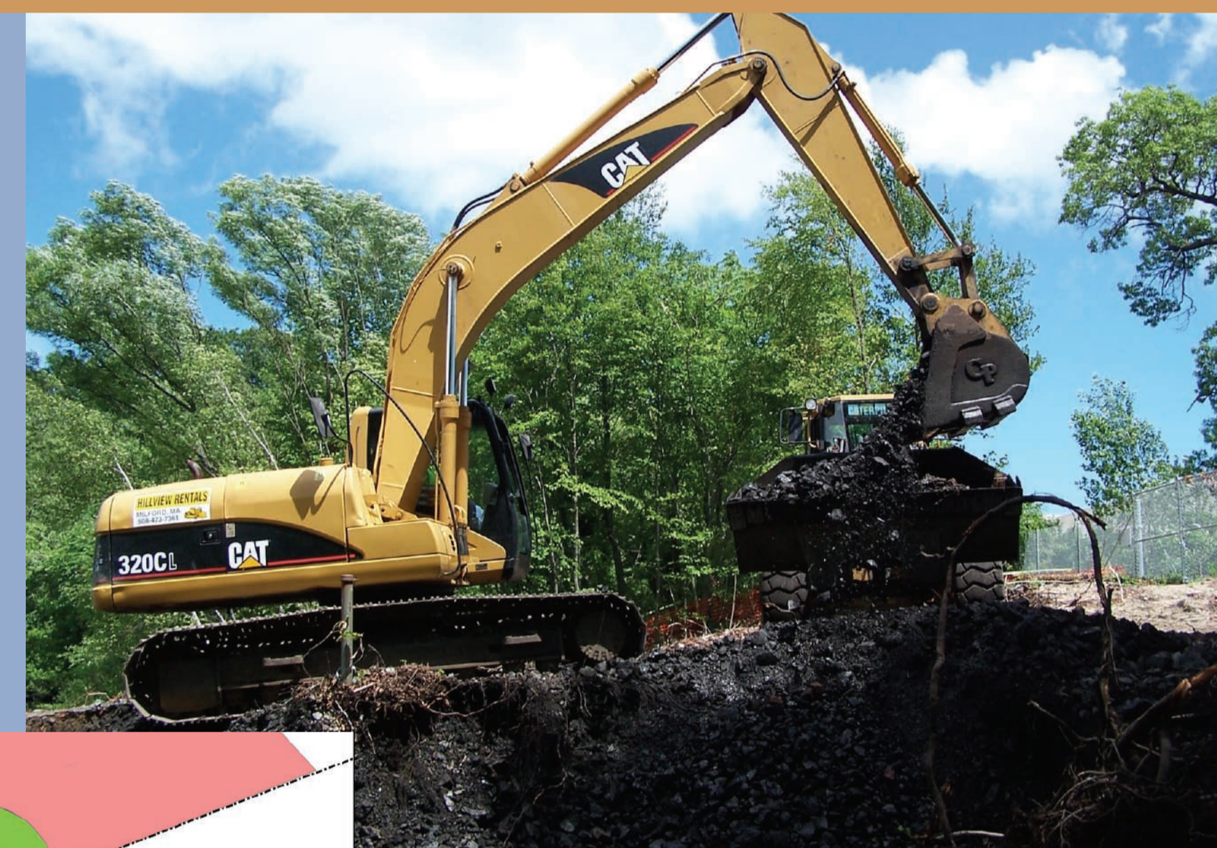
Black slag generated decades earlier as a by-product of Gorham metal-melting operations was removed from this area.
