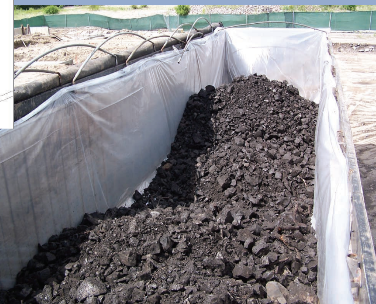
Black slag generated decades earlier as a by-product of Gorham metal-melting operations was removed from this area.
