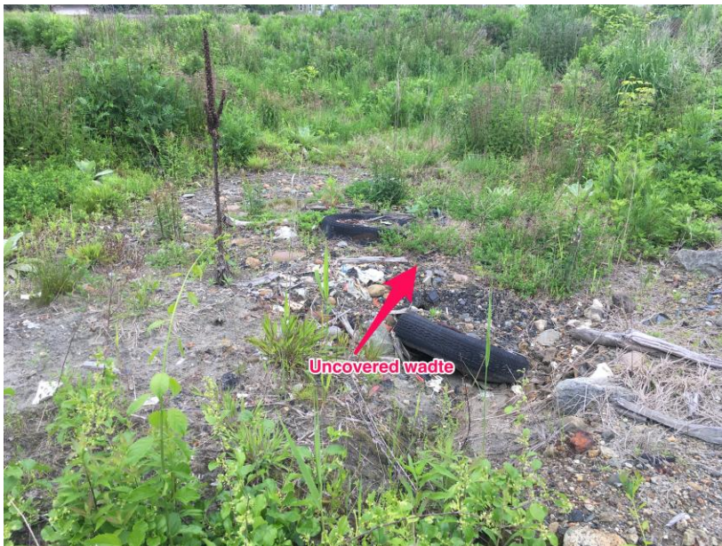
Area in northwest of the site where original fill material is still not covered.
