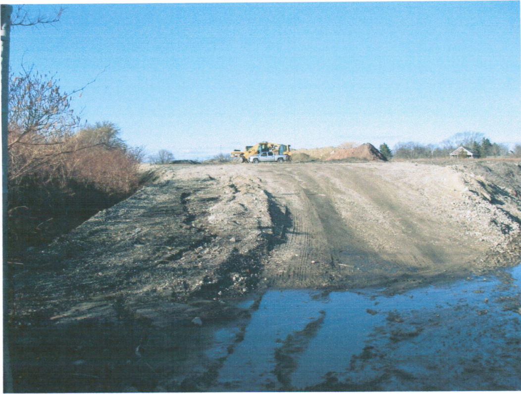
Photo 1 – Site Entrance off Park Avenue
