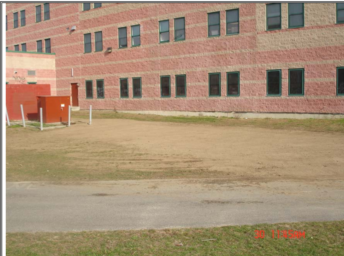
6 | Area near transformer – after filling, 11/30/06.
