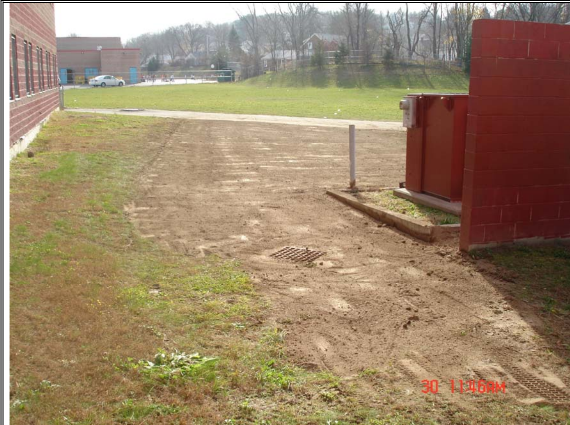
5 | Area near transformer – after filling, 11/30/06.
