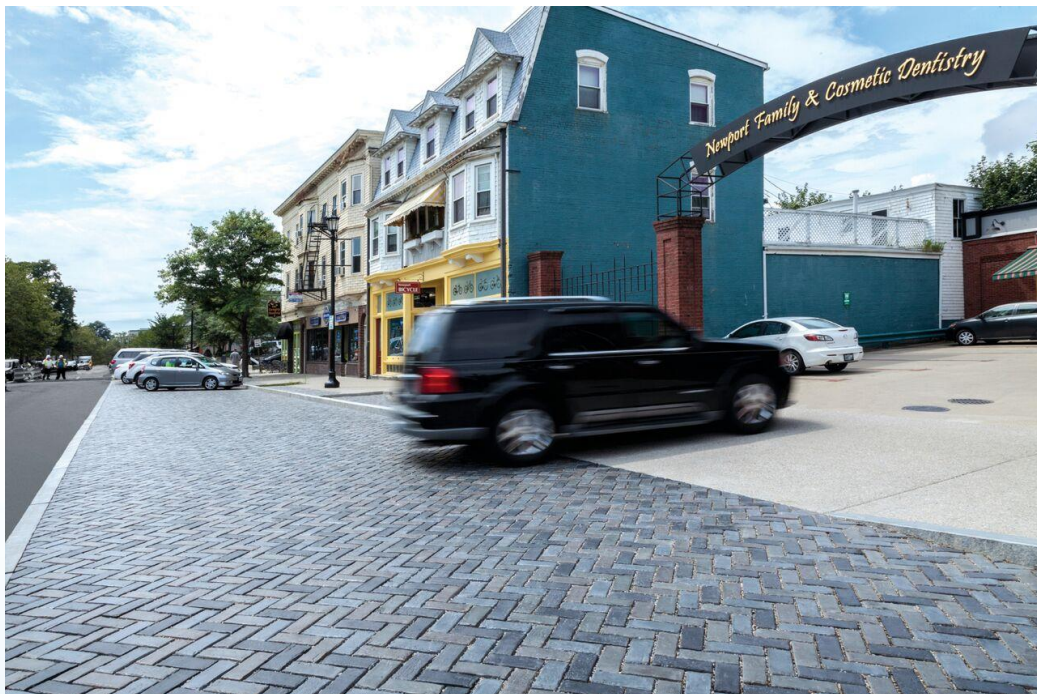
Permeable block pavers on Broad Street in Newport photo courtesy of Unilock New York Inc.
