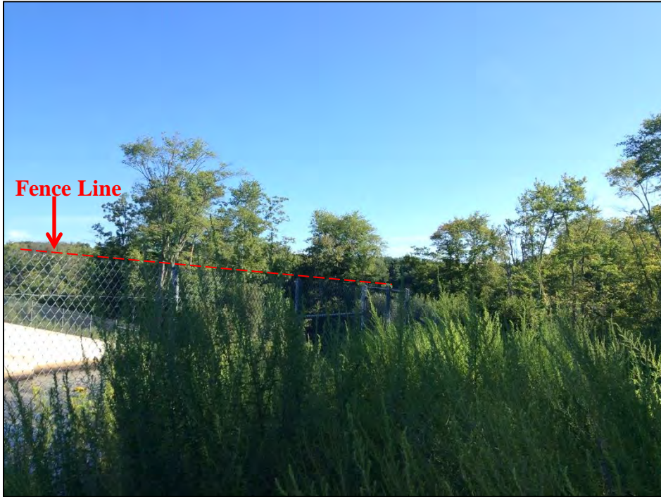
Photo No. 9: The upstream slope right of the primary spillway as viewed from the adjacent waterline right of the spillway approach. Note the heavy overgrowth that prevented inspection.
