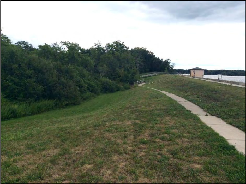
Photo No. 12: The downstream slope as seen from the left abutment.
