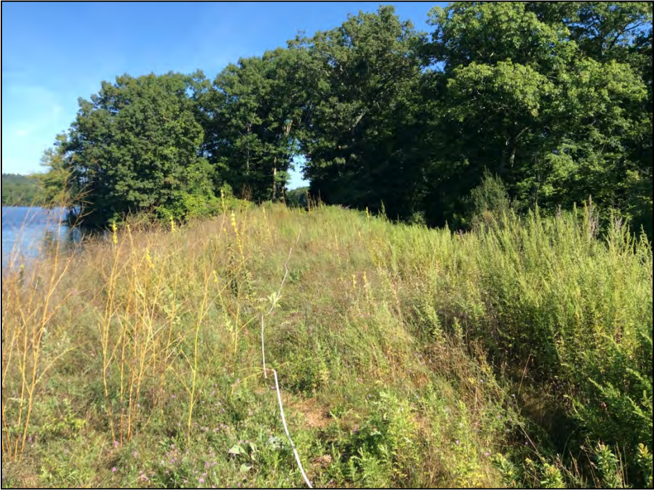
Photo No. 31: Right Dike: The crest as viewed from near station 17+40 looking left.
