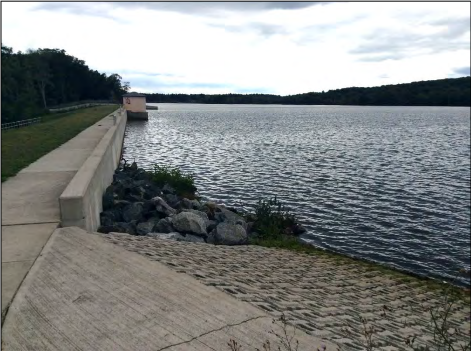
Photo No. 2: The upstream side as seen from the left abutment.
