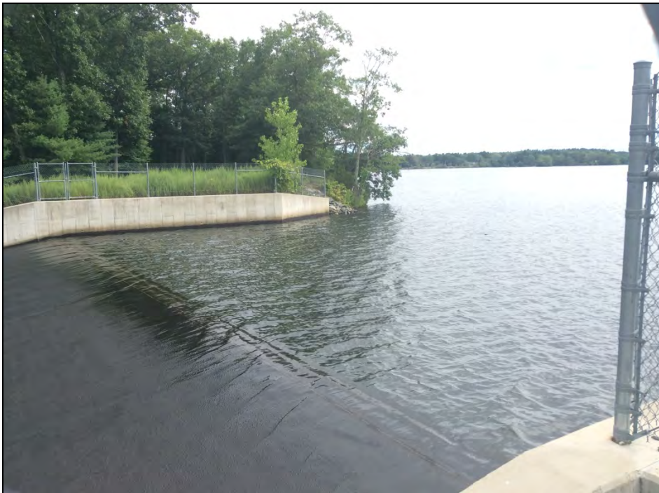
Photo No. 44: The primary spillway approach as viewed from the left looking slightly upstream.
