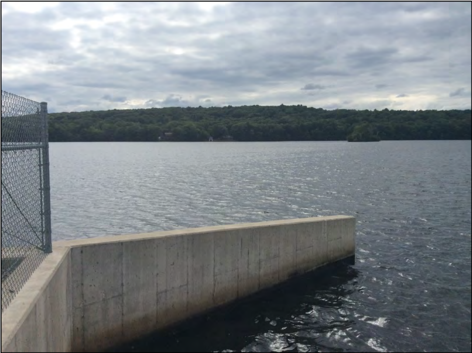
Photo No. 17: An overview of the impoundment as seen from left of the primary spillway.
