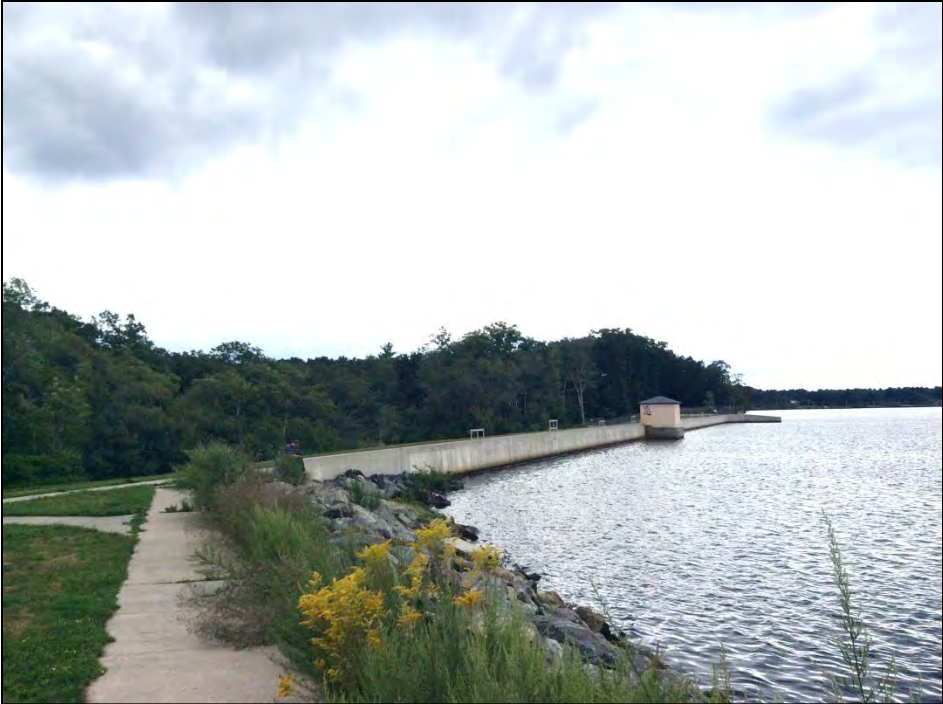
Photo No. 1: An overview of the dam as seen from the Left Dike (beyond the left abutment of the dam).
