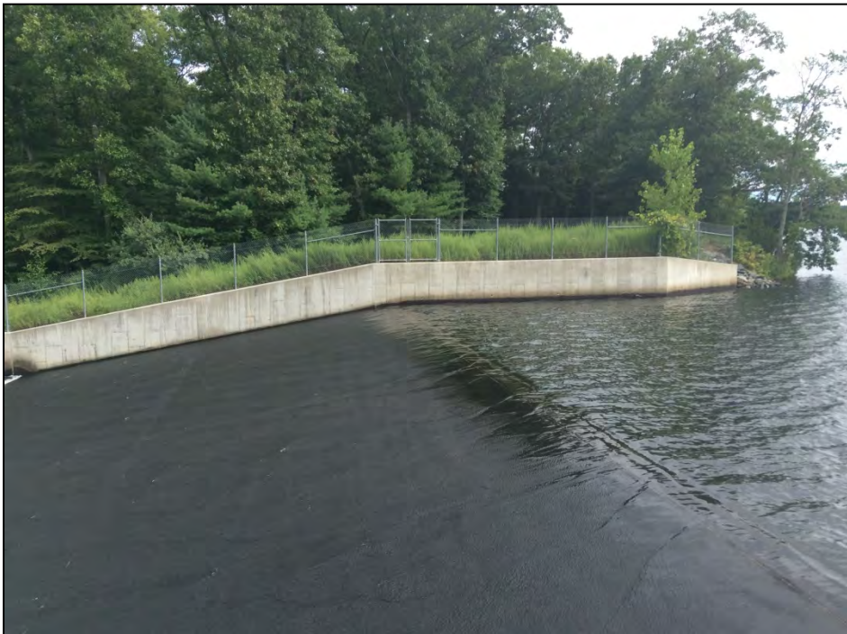
Photo No. 40: The primary spillway weir as seen from the left.
