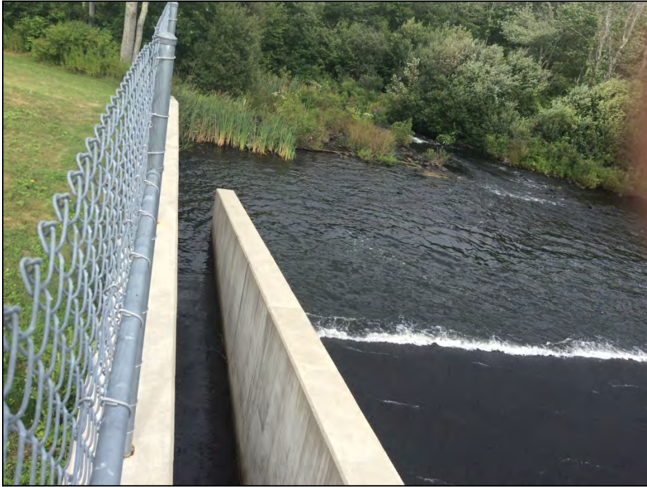
Photo No. 51: The primary spillway by-pass outlet discharge channel looking downstream.
