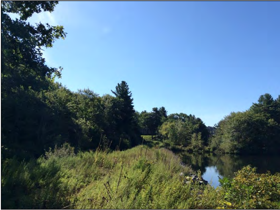
Photo No. 25: Right Dike: Overview of the Right Dike from its left abutment. Note the tall grass and weed growth that prevented a complete visual inspection of the ground surface.
