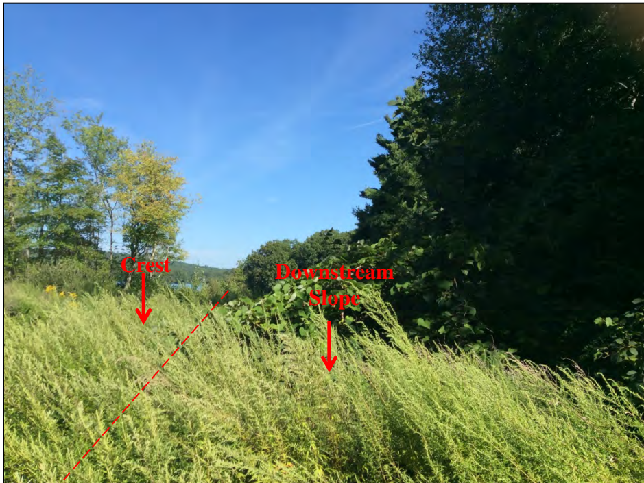
Photo No. 36: Right Dike: The downstream slope as viewed from the right abutment.
