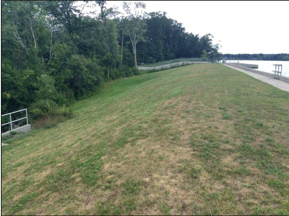
Photo No. 13: The downstream slope as viewed from right of the gatehouse looking right.
