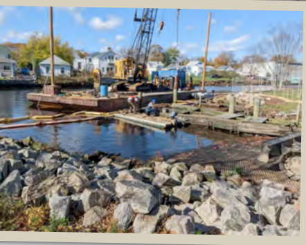
Dock demolition underway at the Main St boat ramp in Westerly.
