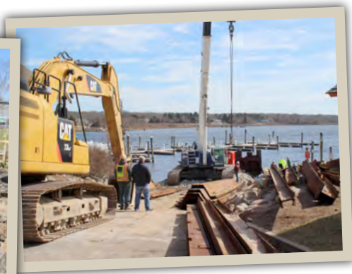
Installing the sheet piling at Marina Park.
