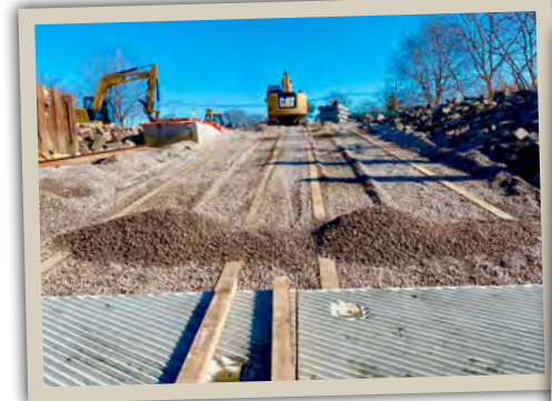
Setting the new ramp slabs.
