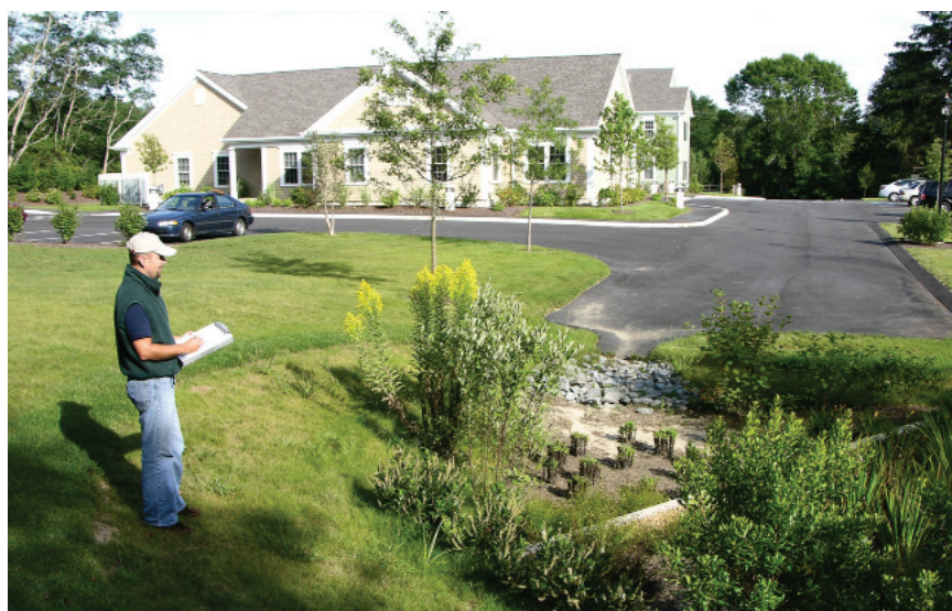
Figure 9-6 Inspection of Bioretention Facility.
