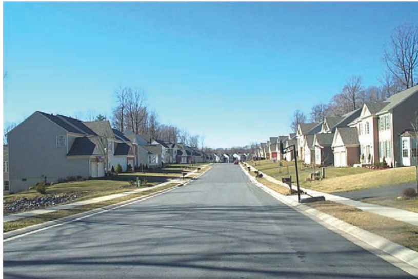
Figure 5-1 Excessive Roadway Design.
