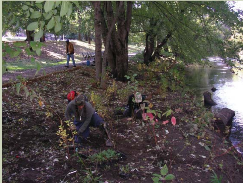
Careful placement and installation of native vegetation is required for restoring buffer areas that were cleared. (HW photo)
