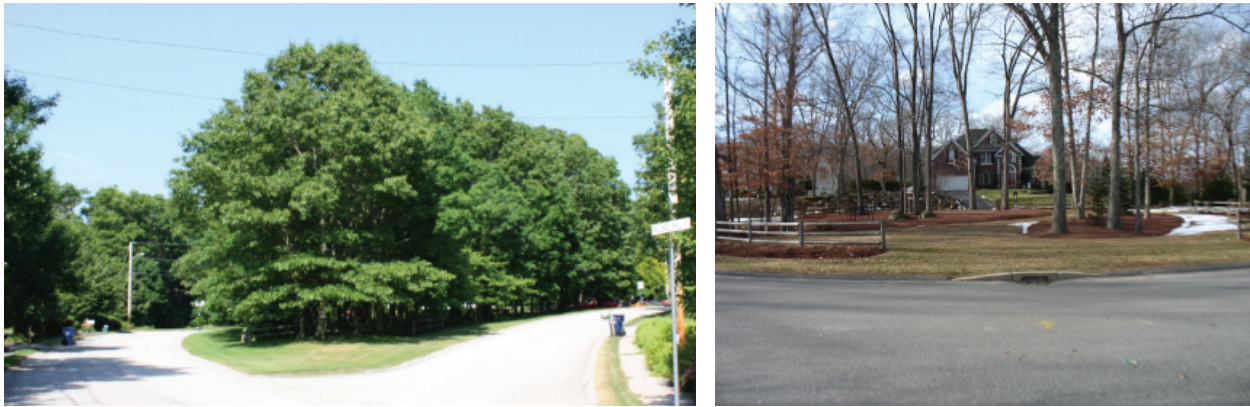
Vegetated cul-de-sacs reduce impervious cover and provide a neighborhood landscape feature. (J. West, left; S. Millar, right)
