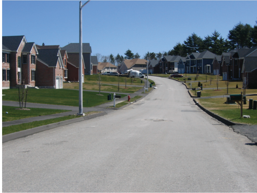
Figure 5-8 Typical Residential Curb Design.
