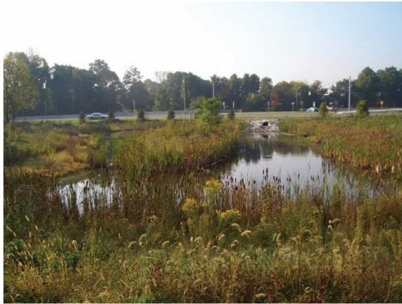
Figure 9-9 Stormwater Facility Requiring Regular Inspection.
