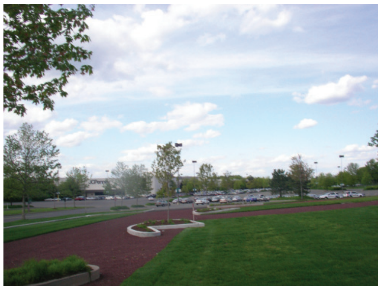
Regular parking areas are constructed with asphalt (background) while overflow areas show pervious travel lanes and reinforced turf in the foreground of this photo. (HW photo)
