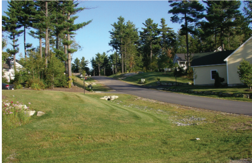
Vegetated swales are used to manage runoff from adjacent roads instead of having typical “curb and gutter” systems. (HW photo)
