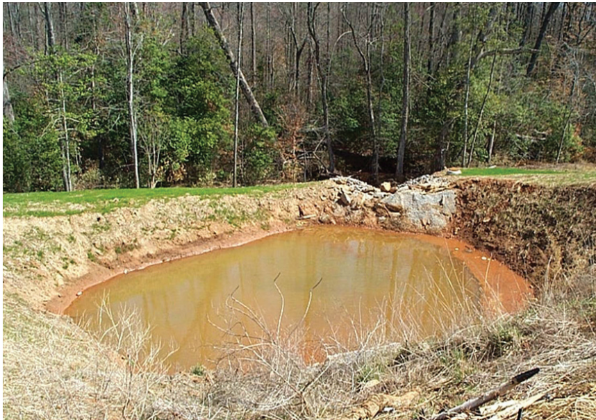
Figure 9-4 Properly Installed Erosion and Sediment Control Practice.
