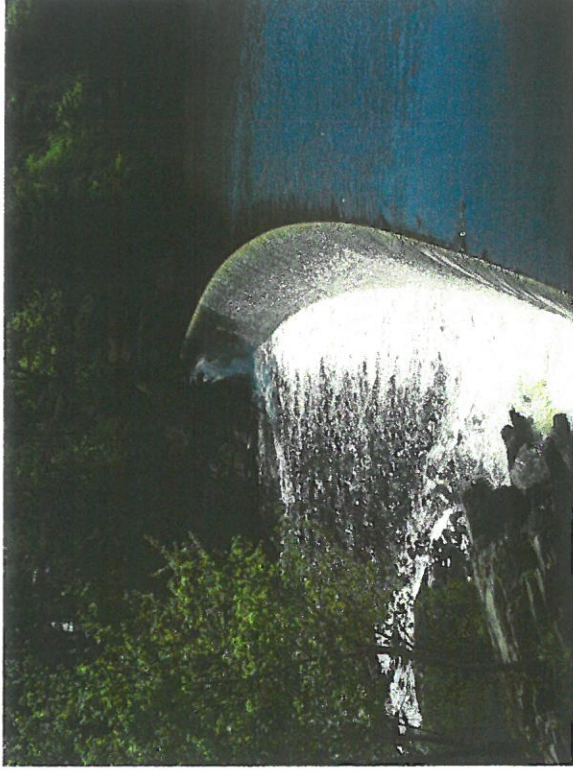
Photo 2. View of the spillway from the left abutment.
