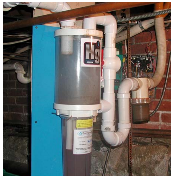
As of July 1, 2008 Rhode Island dentists will be required to install amalgam separators in their facilities.
