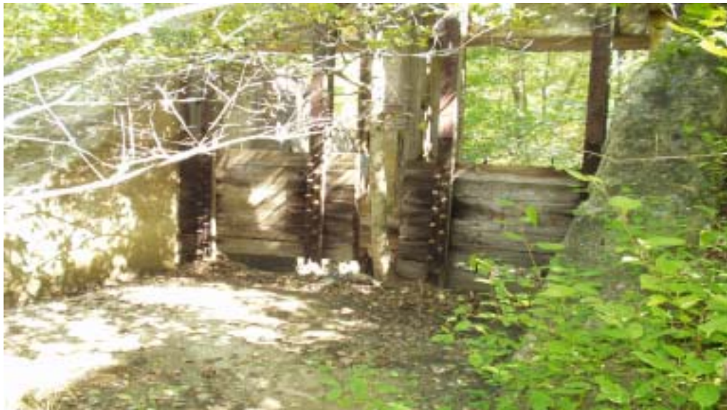
Abandoned gates at Premier Mill Pond Dam (No. 6), Burrillville
