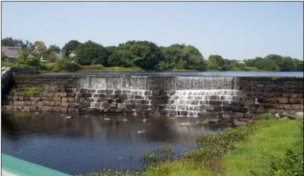
Spillway at Harrisville Pond Dam (No. 8), Burrillville
