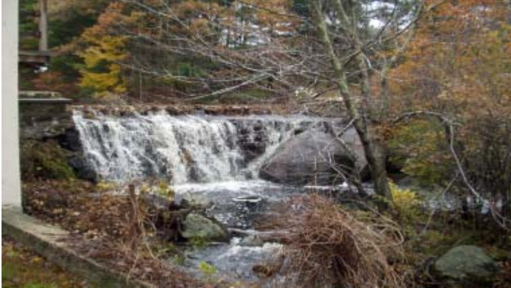
Spillway at Spear Pond Dam (No. 349), Foster
