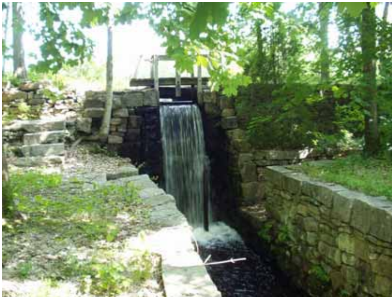
Spillway at Lower Mill Pond Dam (No. 228), Hopkinton
