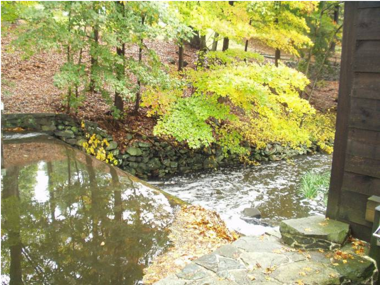
Spillway at Moffett Dam (No. 99), Lincoln
