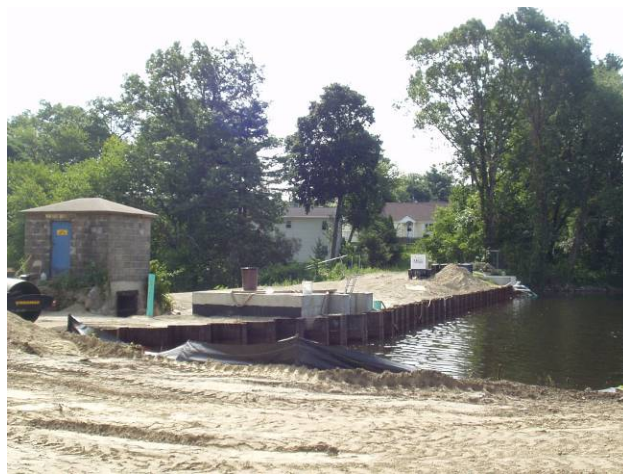
Repair work at Slack Dam (No. 115), Smithfield
