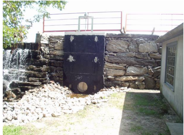
Substantially completed repair work.
