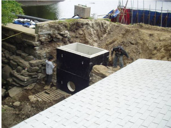
Ongoing repair work.
