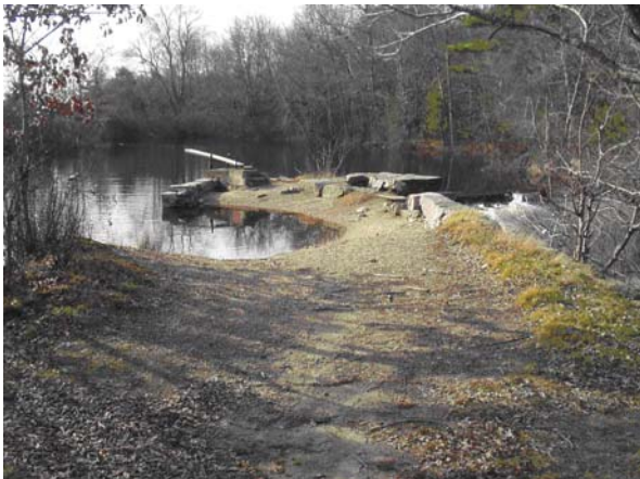
Eroded embankment
