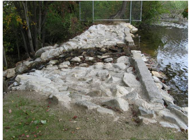
Rebuilt spillway (pond on right)
