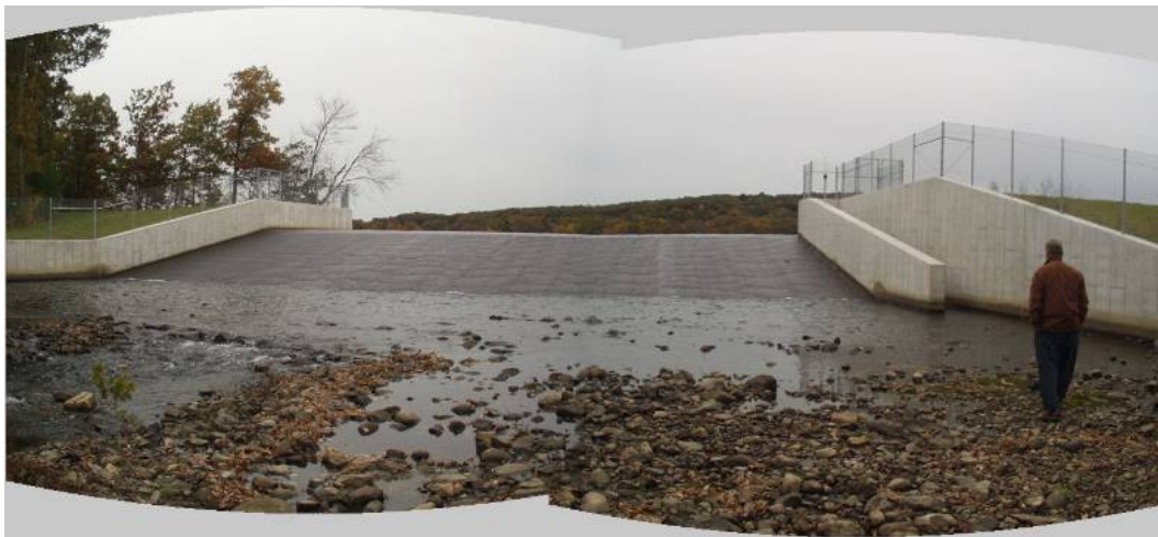
Spillway at Stillwater Dam (No. 108), Smithfield
