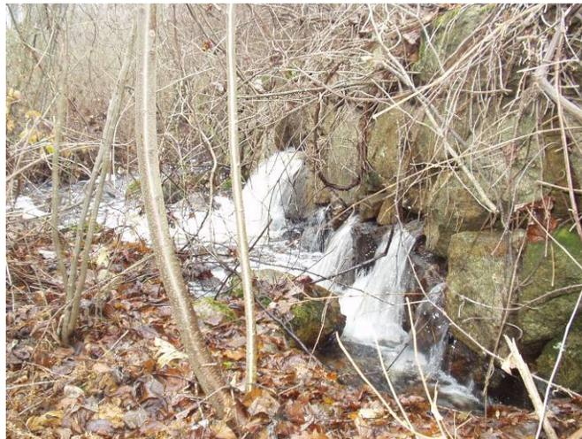
Seepage/leakage at Blue Dam (No. 229), Hopkinton
