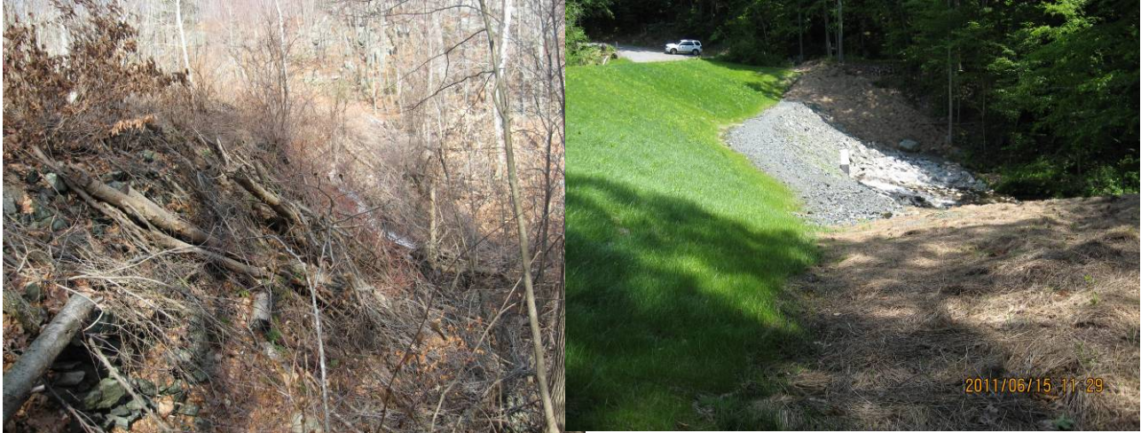
Same view of downstream slope of Limerock Dam (No. 295), Lincoln, before and after work
