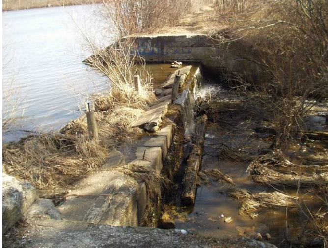
Spillway at Curran Upper Dam (No. 166), Cranston
