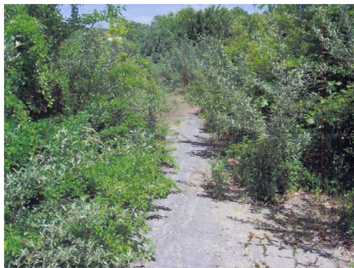
Crest of Stillwater Dam (No. 109) in Smithfield
