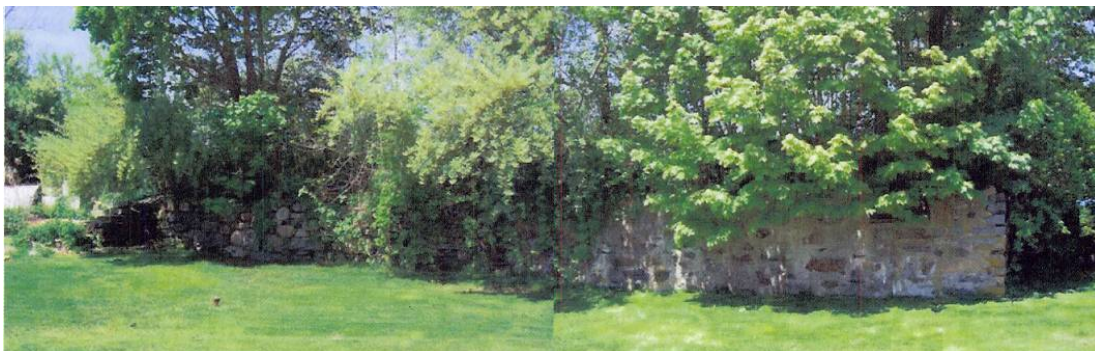
Downstream side of Rodman Mill Dam (No. 615) in North Kingstown.
