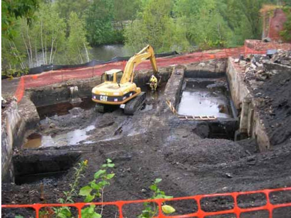
Figure 6. Excavation of the Concrete Tanks Below the Coal Storage Building
