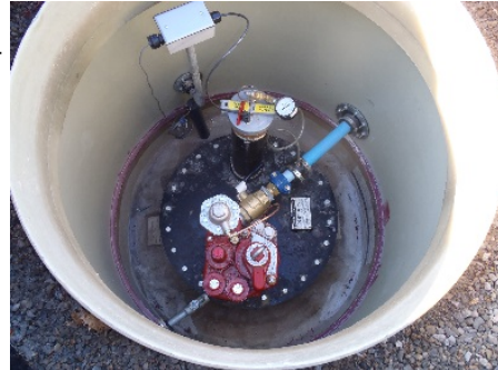
Figure 10 Tank Top Sump
