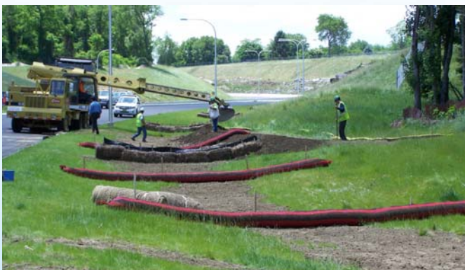
Filter socks used as check dams to control runoff
