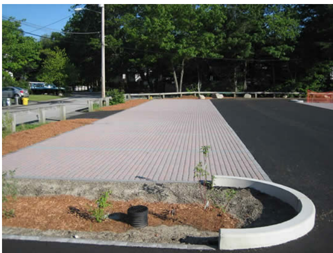
An example of permeable paving. (Source: Silver Lake Project: Massachusetts Executive Office of Energy and Environmental Affairs)
