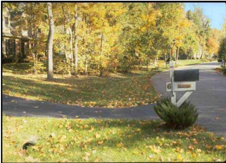
*This development was built using LID. Native vegetation was left to maintain natural hydrology, the road width and driveways were reduced, and road runoff is treated by engineered grass swales along the side of the road*
