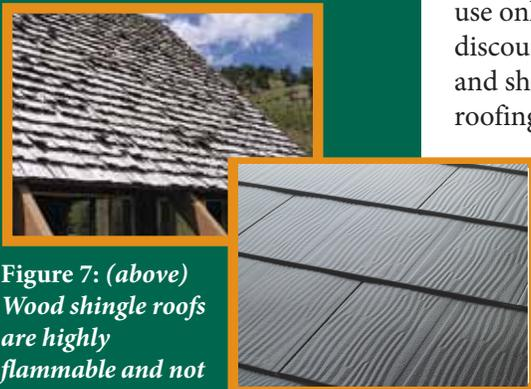
Figure 7: (above) Wood shingle roofs are highly flammable and not recommended. Photo: CSFS
