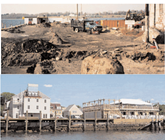
Thames Street Landing, Bristol, before (top) and after.
