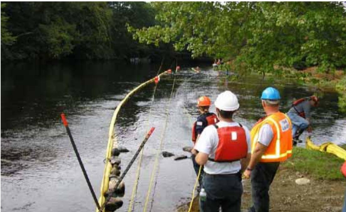
Figure 8. Oil Boom, Deployed to Deflect Oil to a Collection Point
