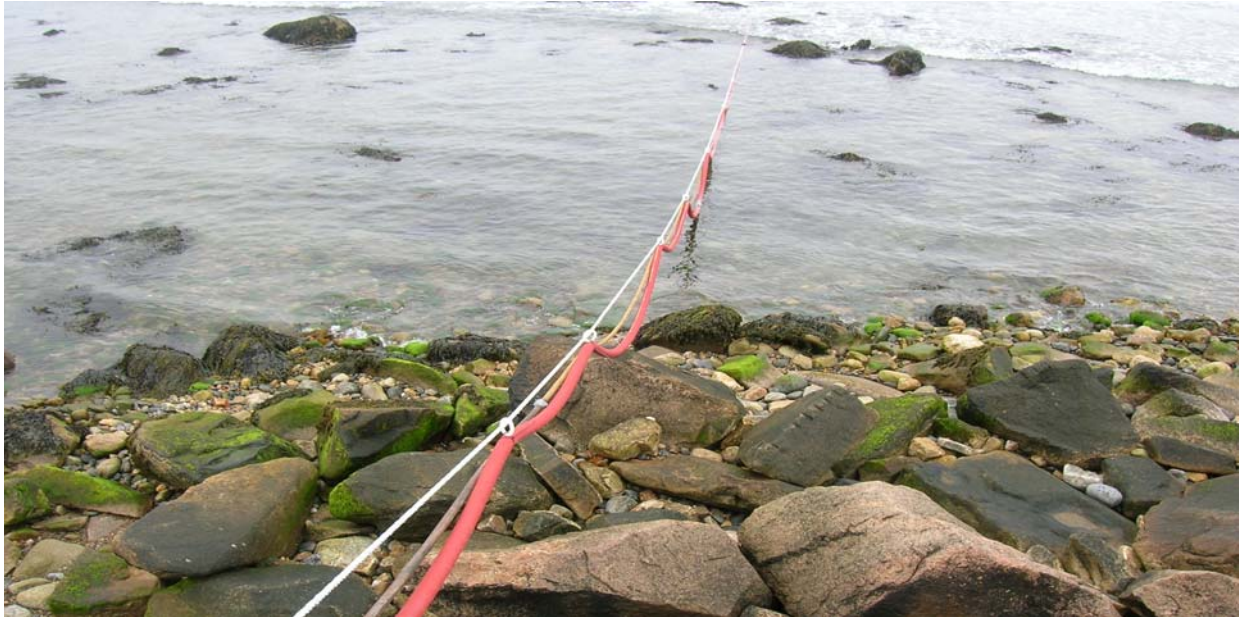
Figure 6. Support line and transfer hose from shore to vessel.
