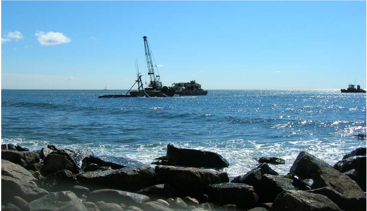
Figure 10. Crane Barge and Tug on scene.
