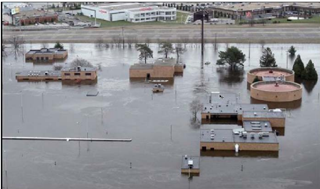
Inundated Wastewater Treatment Facility during the Flood of 2010
