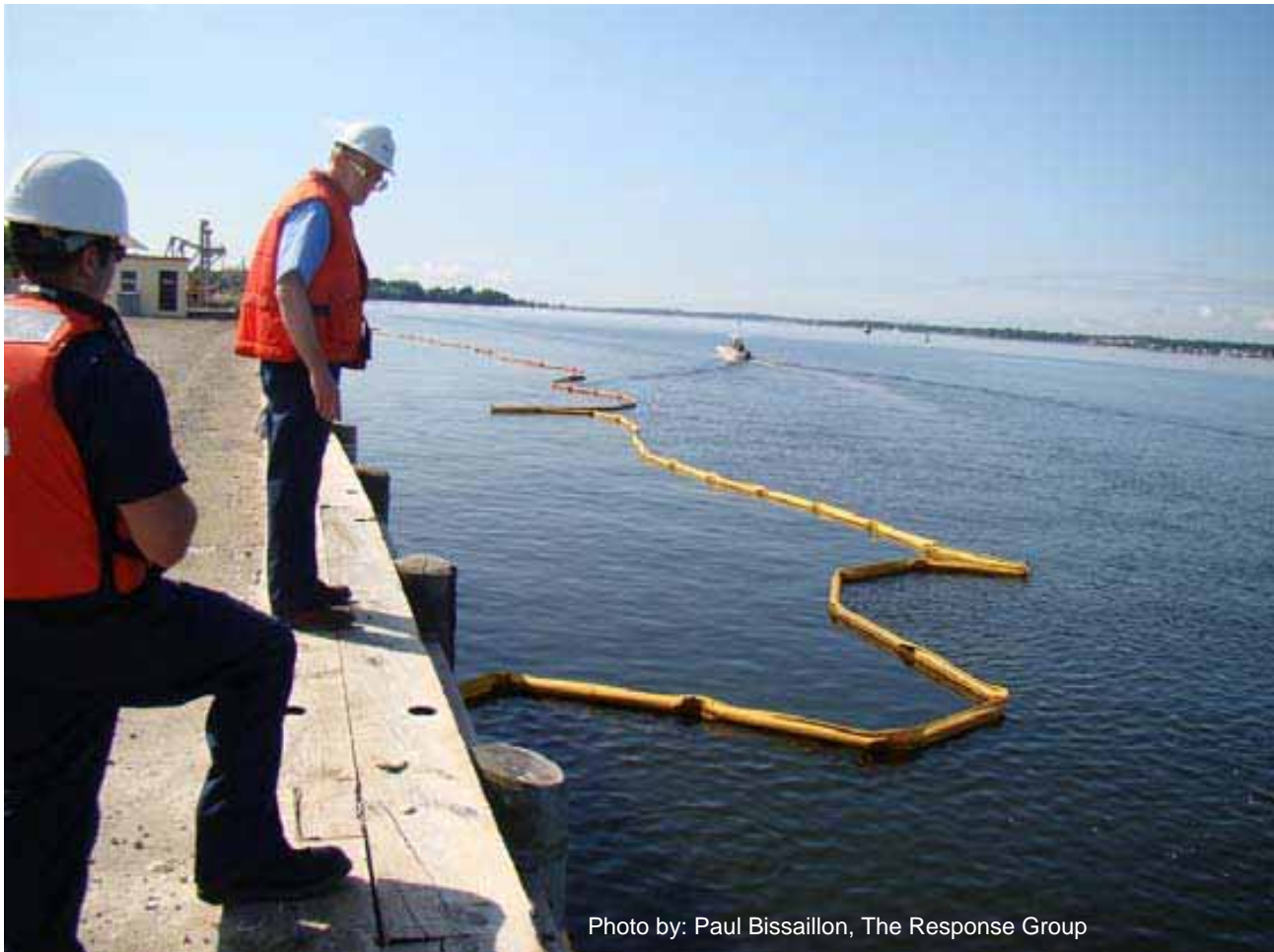
Figure 8 Boom deployment at the northern end of the Exxon Mobil dock
