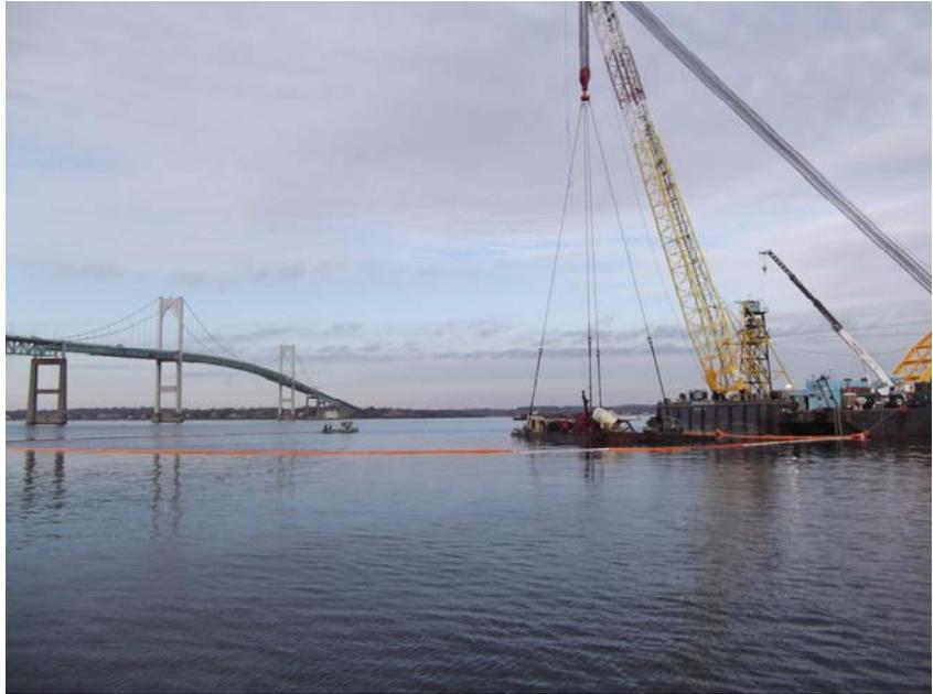
Fig. 7 Boom placement around raised barge to prevent spread of sheening.
