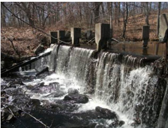
Shady Lea dam removal in North Kingstown
