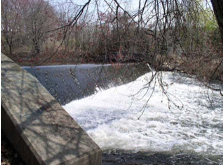
Manton Pond Dam fishway construction in Johnston
