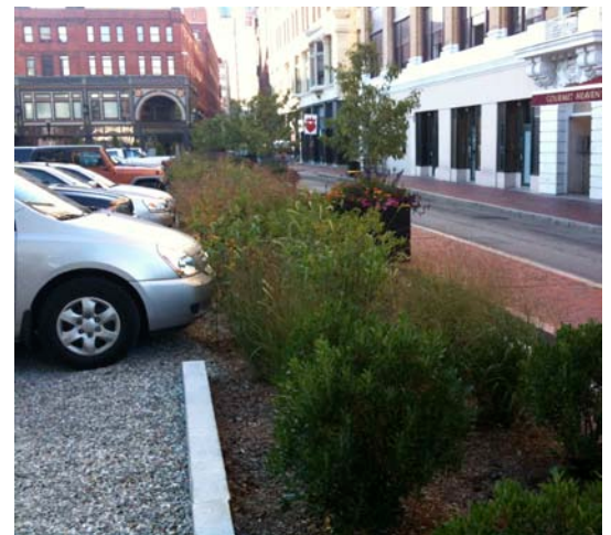
A Providence parking lot retrofitted with low impact development practices to manage stormwater is highlighted in the LID database.
