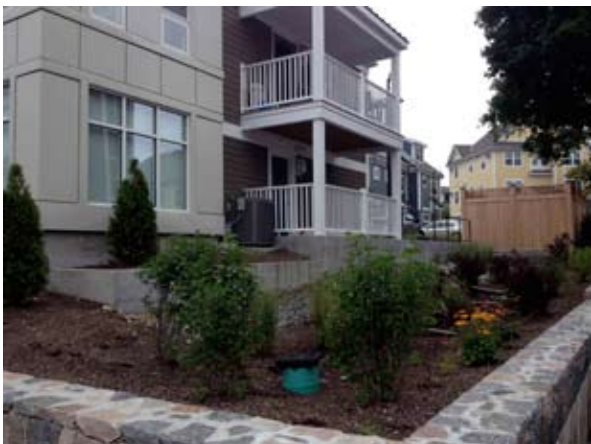
bioswales and bioretention systems are woven into the site design to naturally filter and infiltrate stormwater runoff and save money by eliminating the need for costly underground systems
