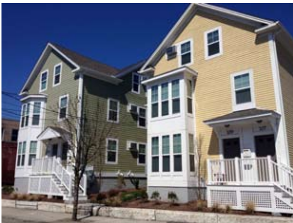
new construction on the "Pope-Manton" site included four new residential and mixed-use buildings along with parking and stormwater management improvements
