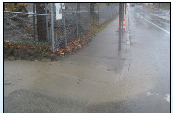
Sediment-filled runoff from a construction site
