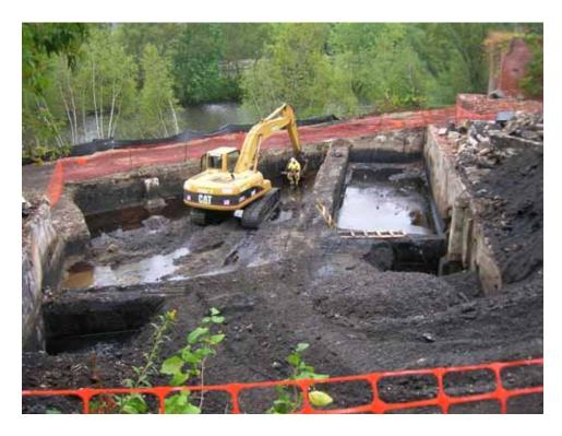
Figure 6. Excavation of the Concrete Tanks Below the Coal Storage Building
