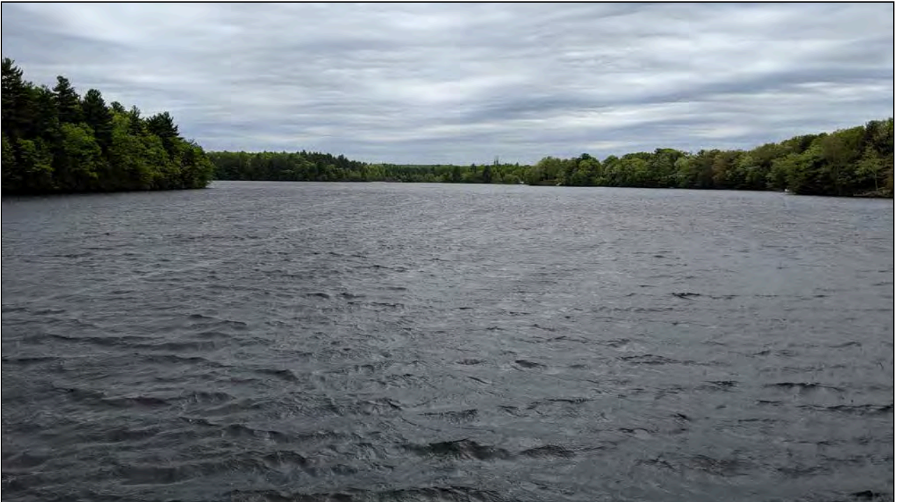
Photo No. 14: Impoundment as viewed from the dam crest above the low-level outlet intake.
