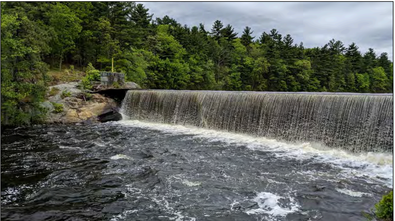
Photo No. 8: Downstream face of the primary spillway.
