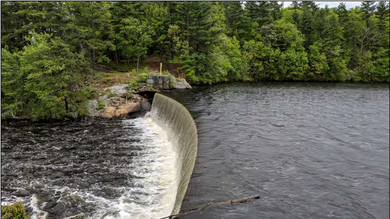
Photo No. 6: Overview of the primary spillway.
