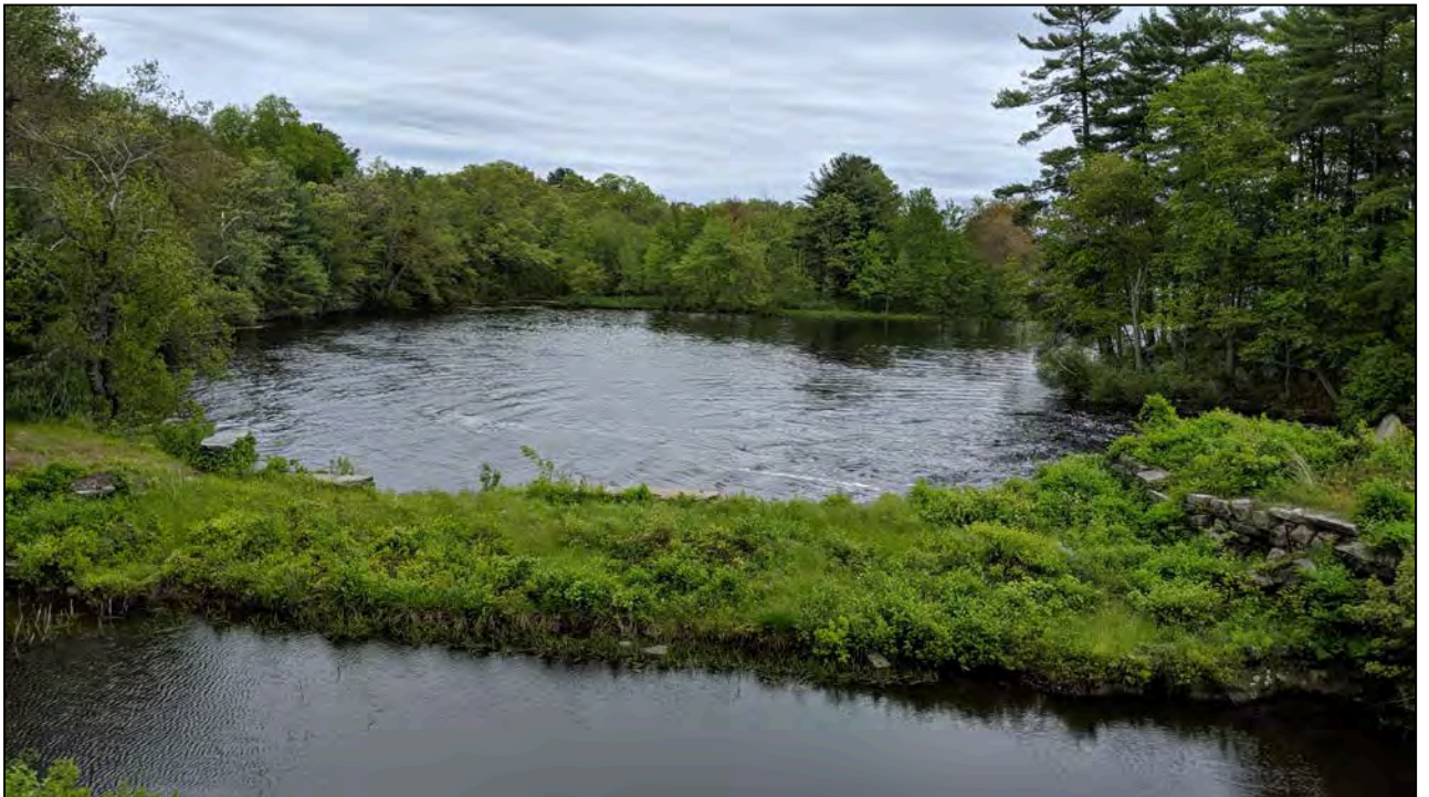
Photo No. 16: Downstream tailwater pond beyond Dam #045. Water in the foreground is the low-level outlet canal.
