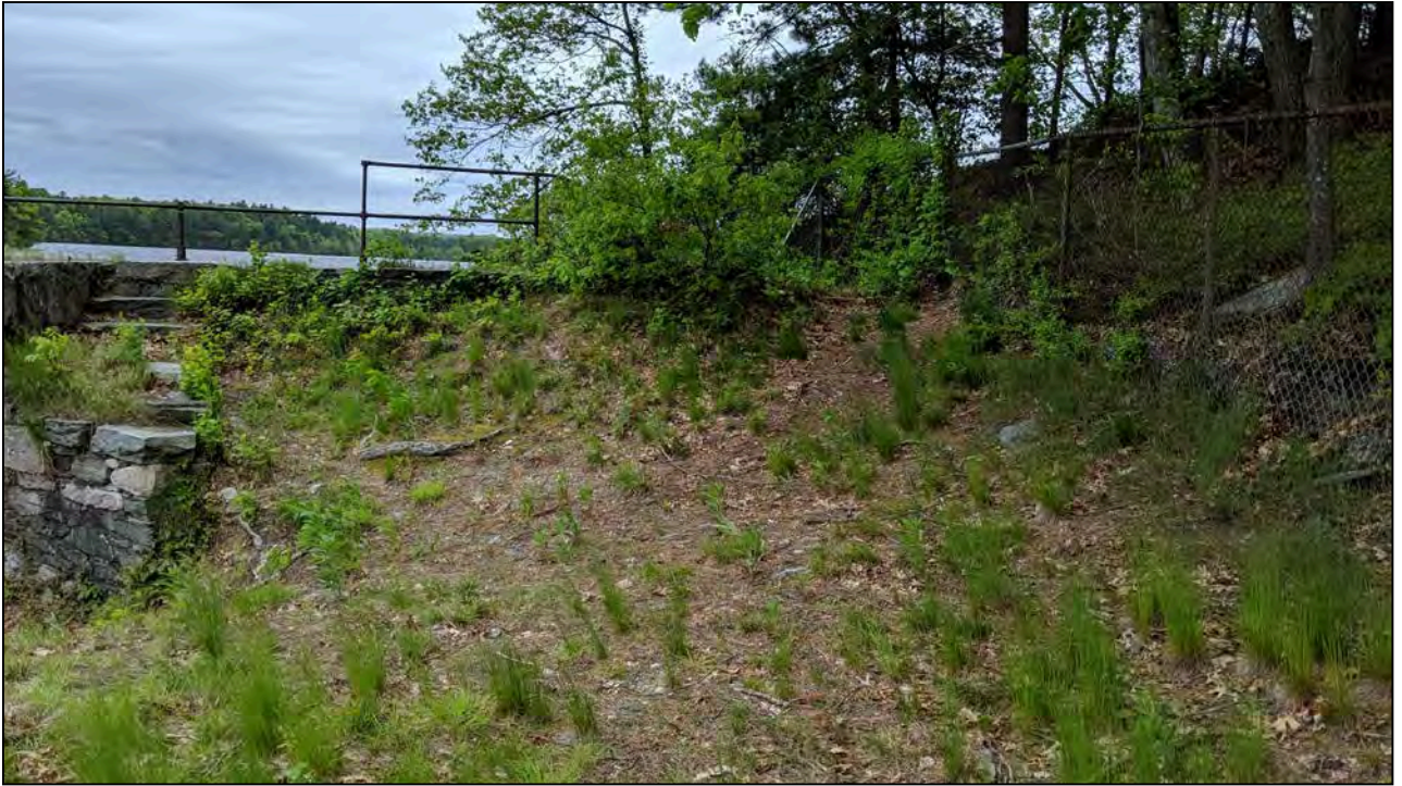
Photo No. 3: Downstream slope between the left abutment and STA 0+30.
